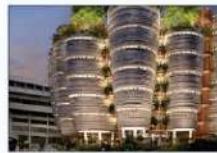
Architect: Heathcote Studio, Learning Hub at Nanyang Technological University, Singapore, 2015
